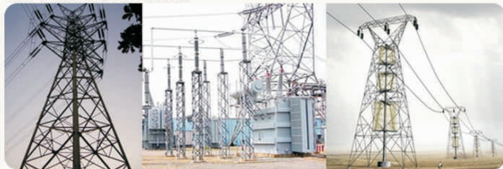
Power Transmission Tower Fabrication
