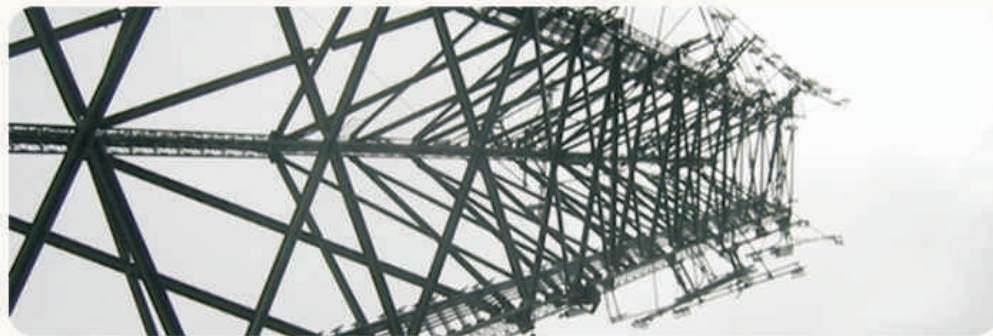
Telecom Tower Fabrication
